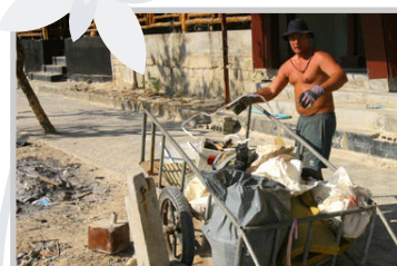
Hard and efficient reconstruction work is in progress in Thailand.
